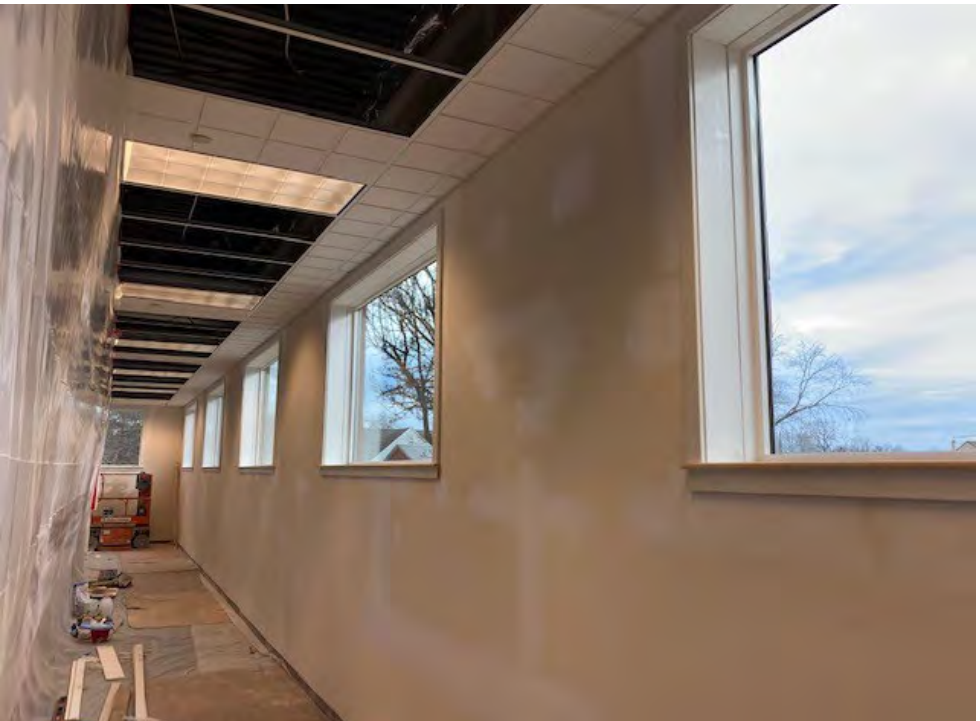
Interior view of west wall with newly installed windows
